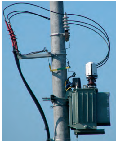
protection of simple transformer station 15/0,4kV
