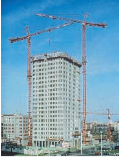
● Crane slewing and Hoisting
